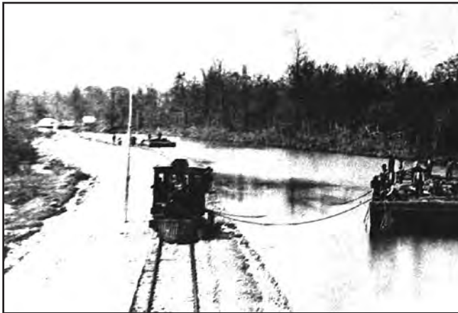
Figure 5. Locomotive towing a barge on Tennessee River between canal locks. (Source: University of North Alabama, William Lindsey McDonald Image Collection)
