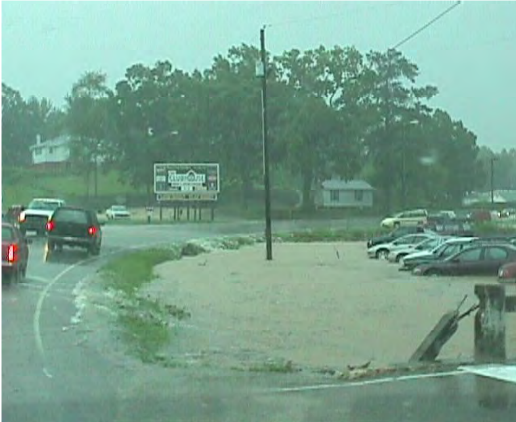
Highway 13 After Storm Event
