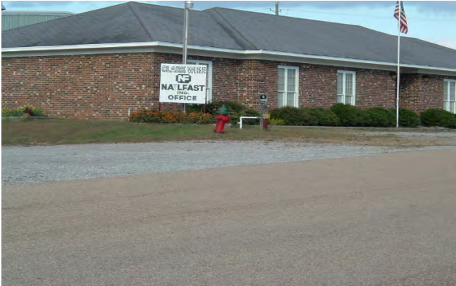
Nailfast Office Botush Industrial Park
