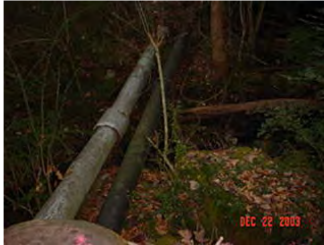
Old Gravity Sewer at Creek Crossing
