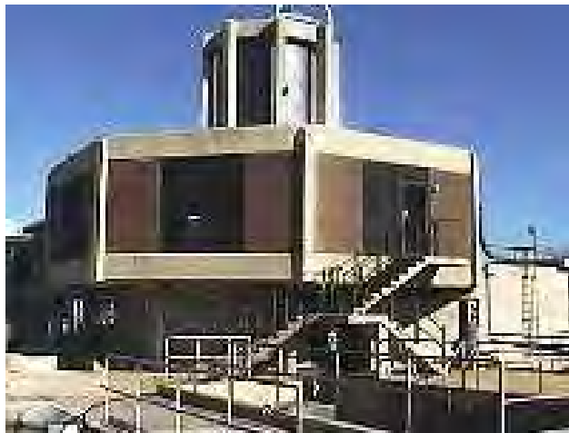
Upper Bear Creek Water Filter Plant
